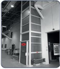
The Mastlift is fitted with our freight elevator control which includes autolevel system and soft start / stop.
